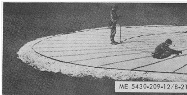
Figure 8-21. Tightening bolts in tank bottom.
