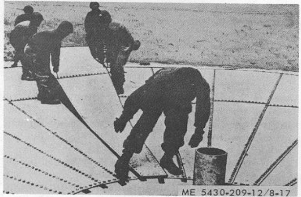
Figure 8-17. Checking Bolt spacing at installation of last bottom section.
