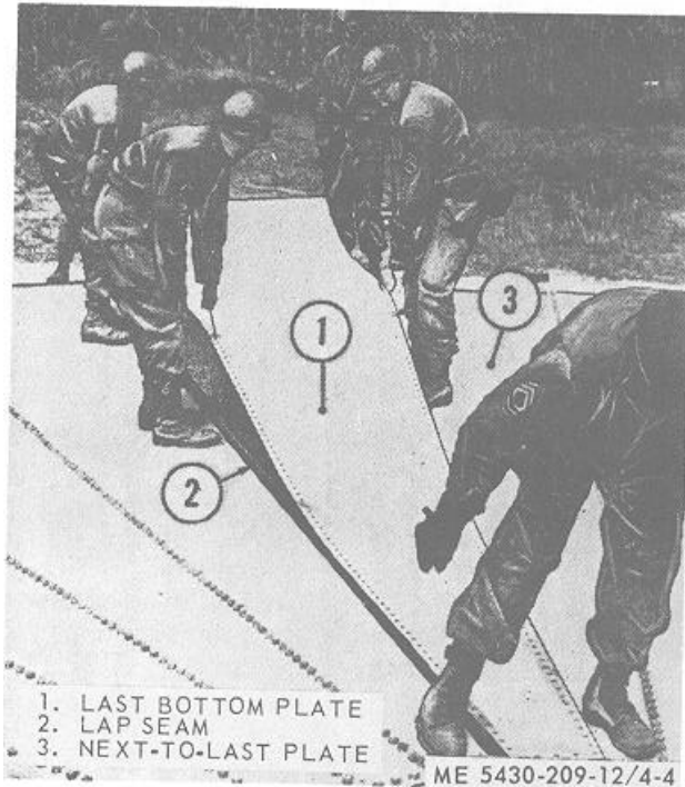
Figure 4-4. Checking bolt spacing at installation of last bottom plate.
